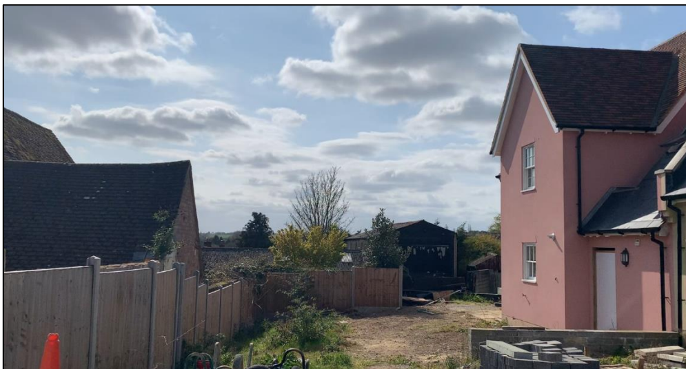
figures 3: Images of the existing dwelling on plot 6
