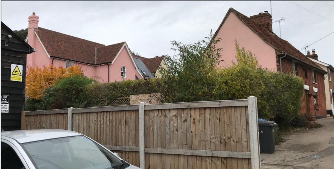
figure 31: View Towards White Horse House from Pilgrim's Garage with 'as-built' dwelling on plots 6 intruding from behind
