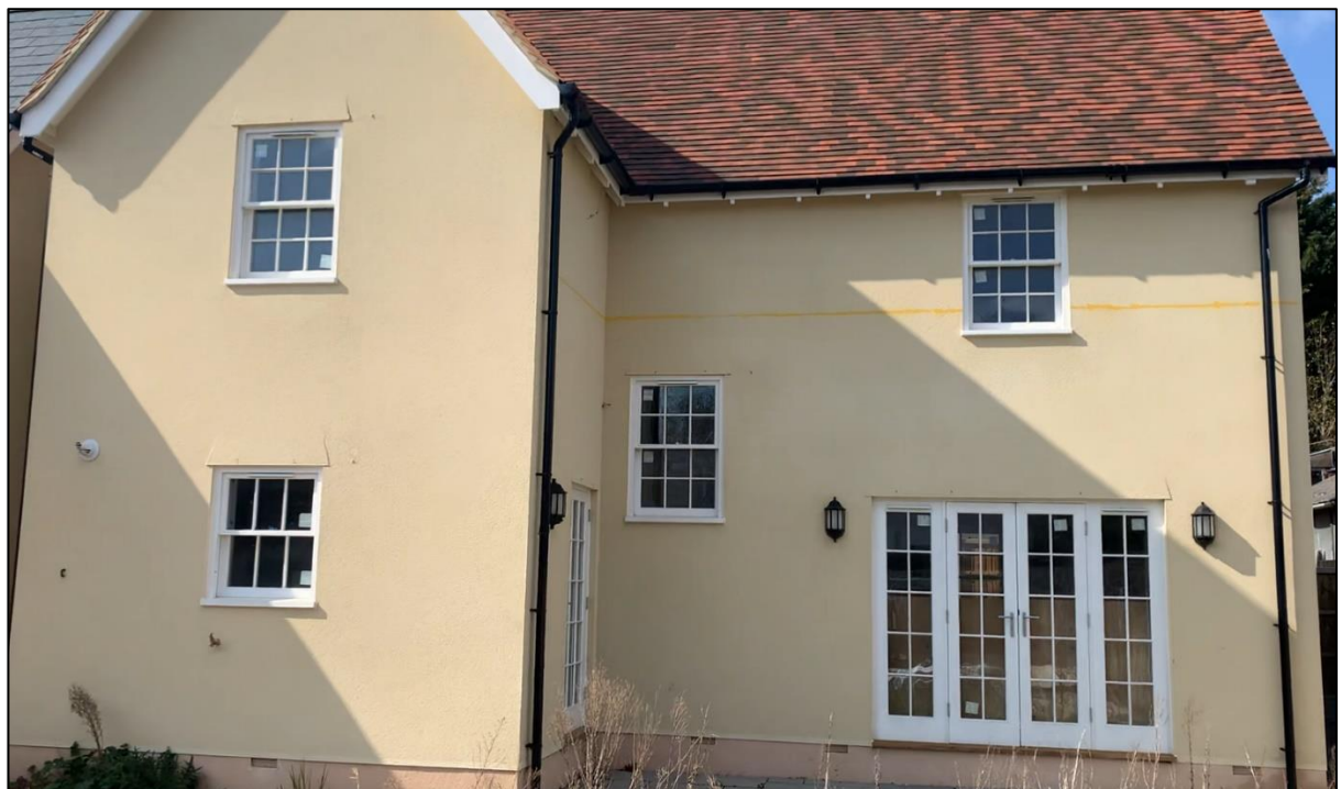
figures 2: Images of the existing dwelling on plot 5
